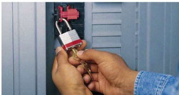
Circuit Breaker Lockout
