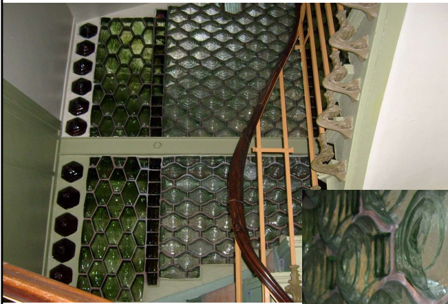
Glass block wall and detail of the blocks.
