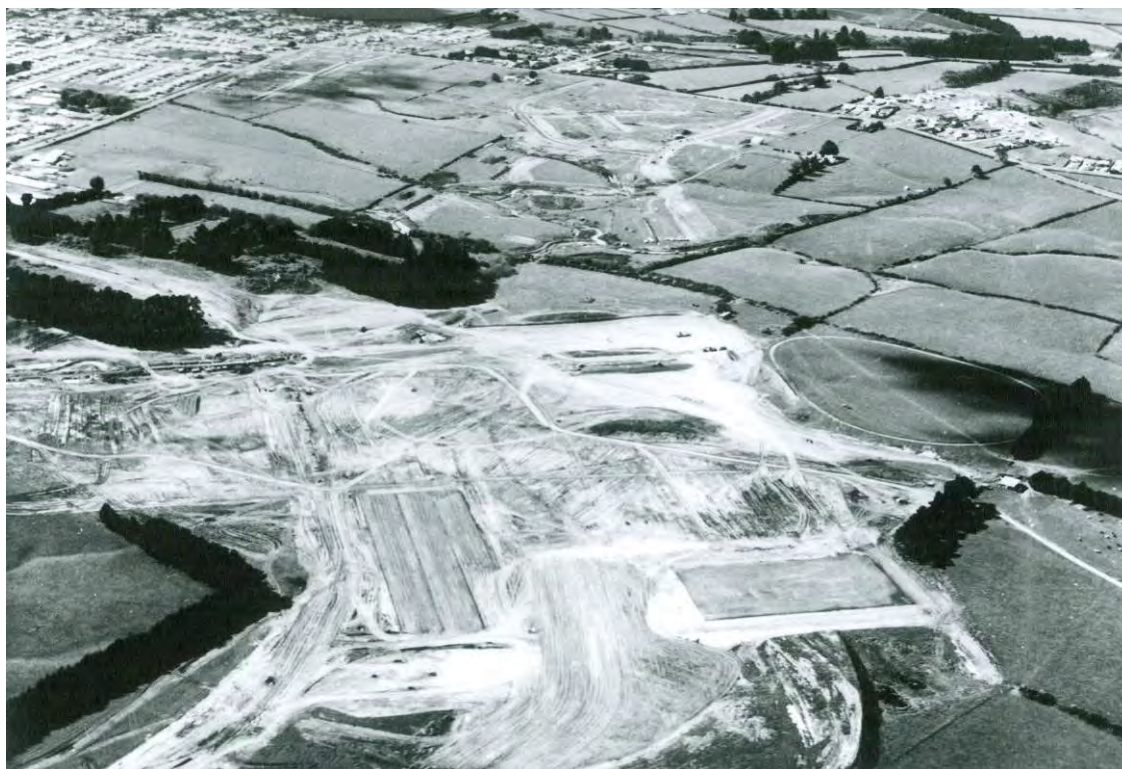
Figure 27: Forming the site of the Mangere town centre, c.1970. Source: Penman Collection, Manukau City Libraries, MGE III, 1, 30.
