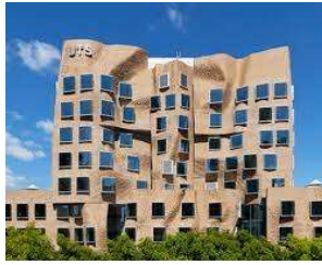
Dr Chau Chak Wing Building 2015 Sydney UTS
