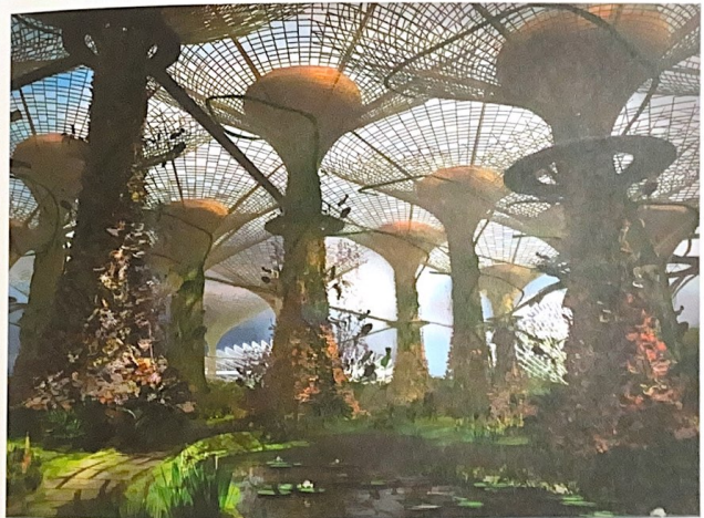
At the heart of the gardens are the Supertrees—a fusion of nature, art, and technology. The spectacular vertical tropical gardens feature ferns, orchids, and climbers as well as environmental engines for the gardens, equipped with photovoltaics, solar thermal collectors, rainwater harvesting devices, and venting ducts.
