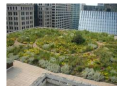
Chicago City Hall – Green roof
