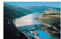
Clyde Dam, South Island, NZ
