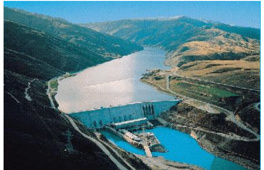
Clyde Dam, South Island, NZ
