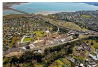
Waterview Tunnel under development
