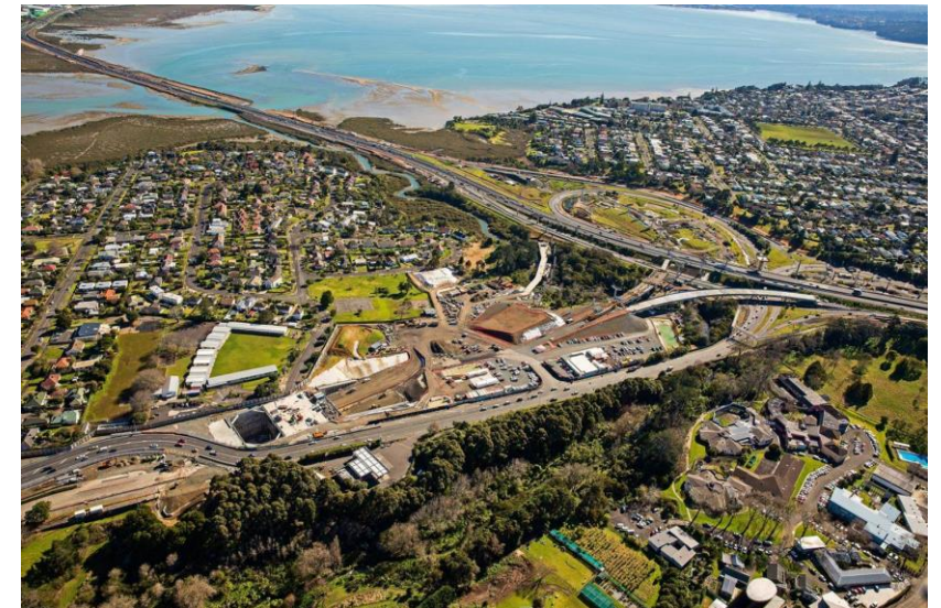
Waterview Tunnel under development
