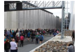
Waterview Tunnel, photo kindly shared by Ray Chang, 2020
